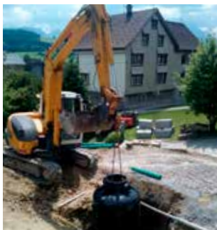
Installation des Wassertanks
